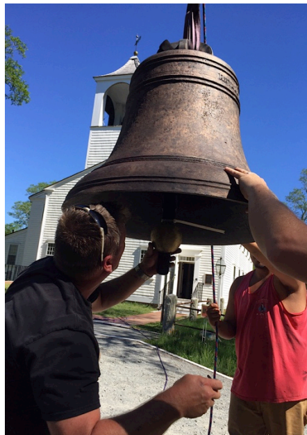
The photo at left shows the bell arriving with yoke and clapper attached. Both needed to be taken off the bell for it to fit into the tower. Photos at right show the new yoke and clapper.
