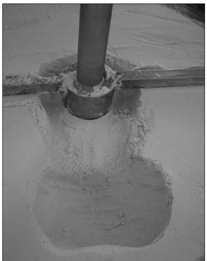
Figure 18. Puddling hole prepared for the pour.
